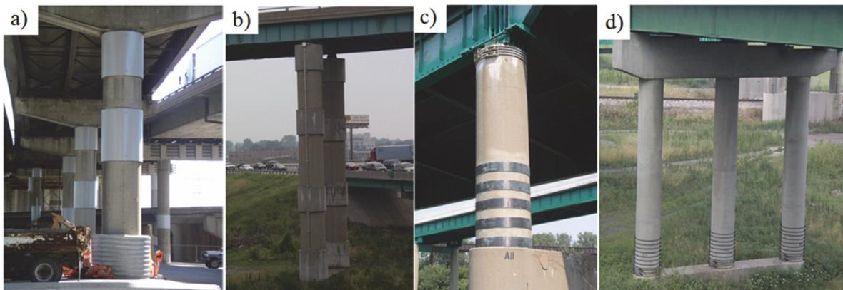
Fig. 7.1 Pier retrofit with: a) steel jacket; b) concrete overlay; c) CFRP strips; d) post-tensioning (Padgett 2007).
