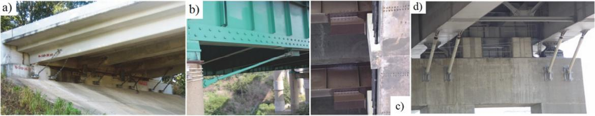
Fig.7.2 a) Retrainer cable bar; b) retractor bar; c) bumper block; d) shock transmission unit (Padgett 2007).
